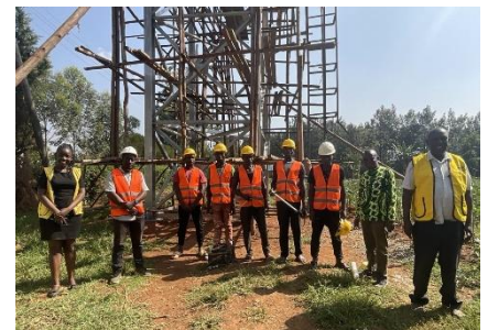
Contractor Crew Infront of Water Tower
