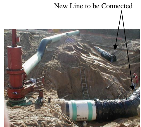
Figure 15 Plugging machine and bypass in operation
