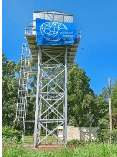
Water Kiosk Tower Completed
