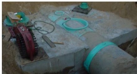
Figure 14 Tapping fittings and thrust block
