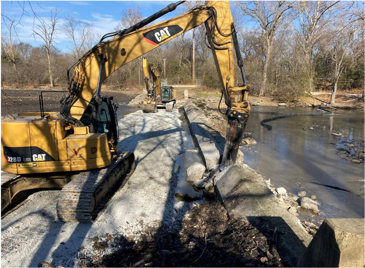
Removal of the Low Head Dam at Graue Mill 2023, MWRD photo
