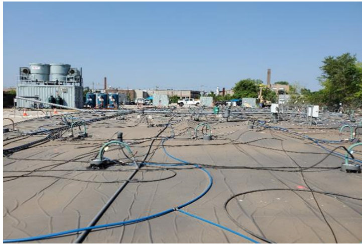
Electrical Resistance Heating (ERH) remediation. Credit – V3 Companies, Ltd.
