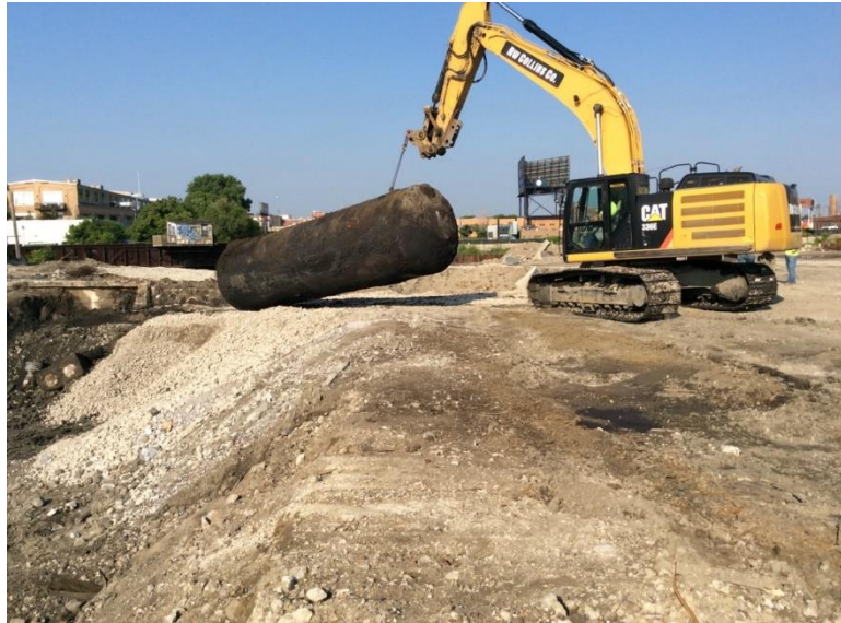
Underground storage tank (UST) removal. Credit – V3 Companies, Ltd.
