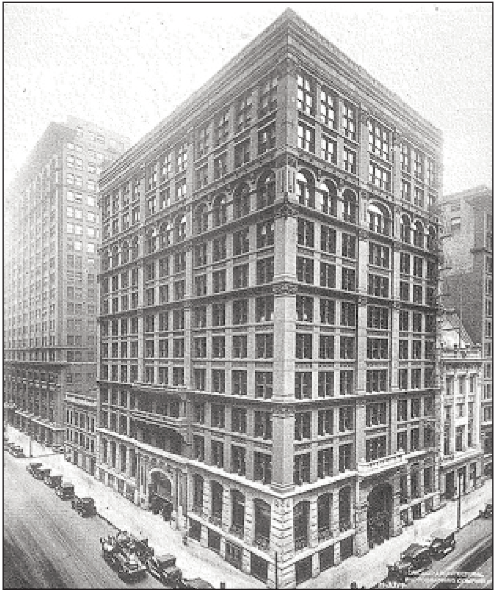
The Home Insurance Building with its steel and iron frame was calculated to weigh only one third as much as a heavy masonry building the same size. This extraordinary design allowed for larger windows and a modern exterior. Photo by City of Chicago Department of Planning & Development, Landmarks Division.
