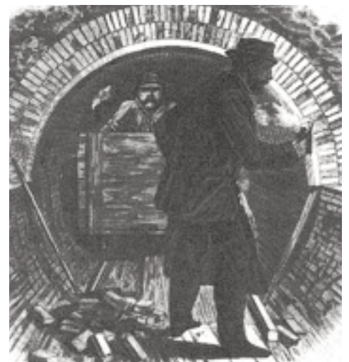
Construction of Chesbrough's brick lined tunnel.*
