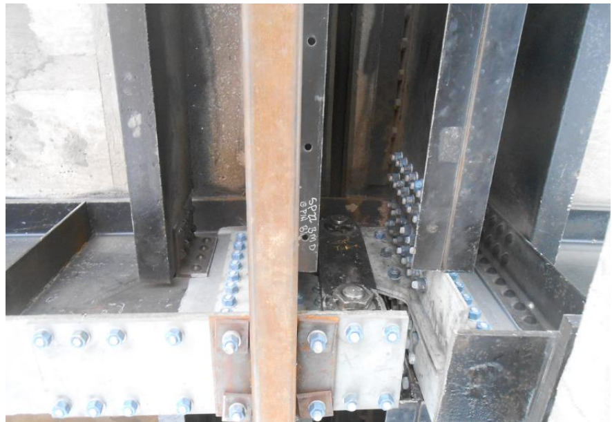
Figure 1: Repaired Pin and Link Joint with Temporary Shoring Shown (As viewed from below)
