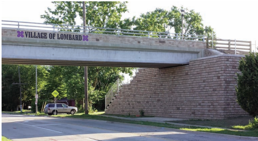
Great Western Trail GRS-IBS structure over Grace Street in Lombard, IL
