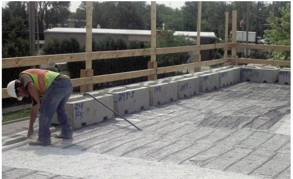
GRS construction for the Great Western Trail project in Lombard, IL.
