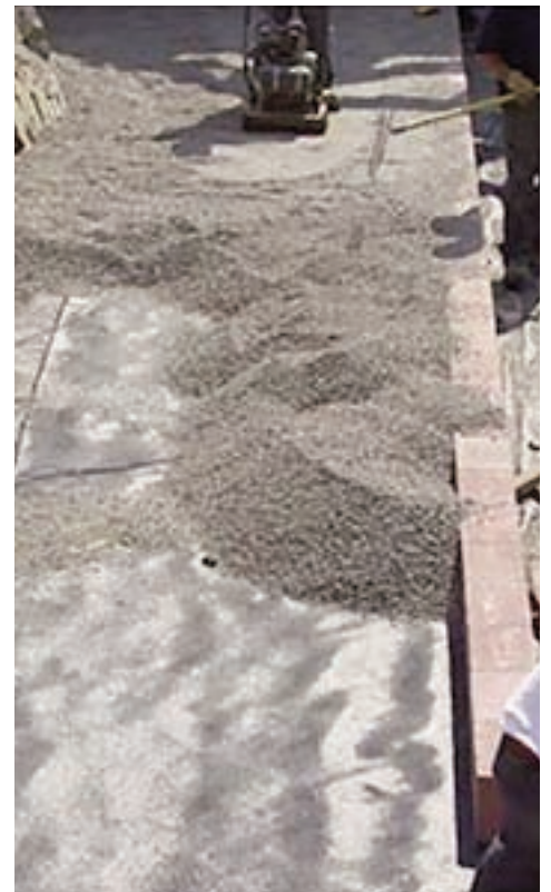
Typical GRS construction showing modular blocks, granular fill, and geotextile fabric.
