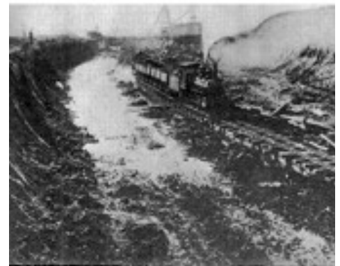
Two construction photos of the Illinois and Michigan Canal during the 19th Century. Original caption for left photo - "Excavation in Earth for Drainage Channel and Waterway One Third Depth".
