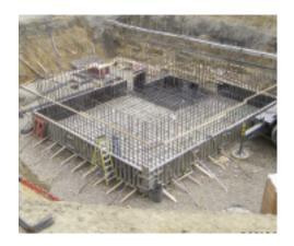
support this structure, due to the presence of thick fill soils with inconsistent bearing capacity. Also, displacement piles were required, because much of the fill soil was mine waste that could not be moved, in order to stay in compliance with the mine permit.
